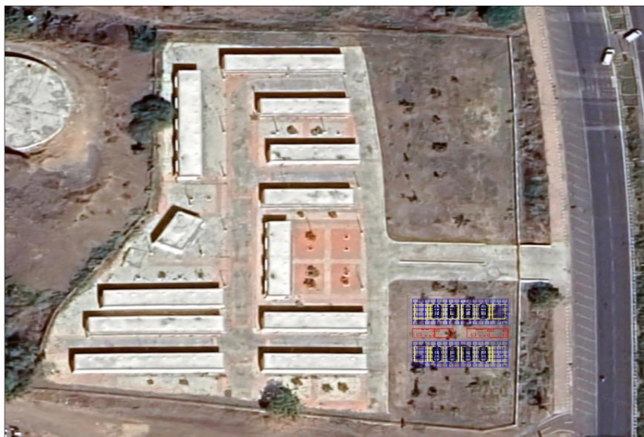
Figure 1: Site for setting up solar carport at SoU
