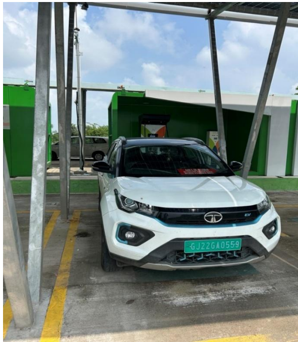
Figure 8: EV charging at SoU site
